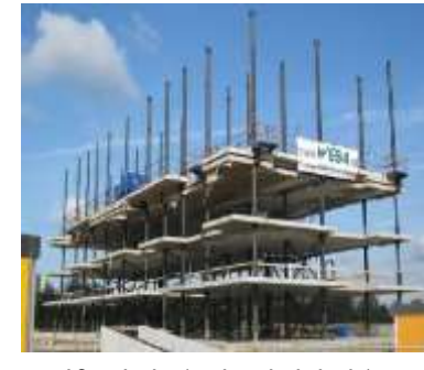
Lift slab (/ jack blok)
