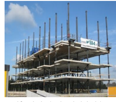
Lift slab (/ jack blok)
